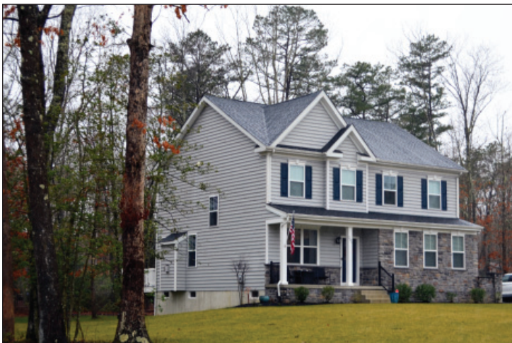
Above: The housing development above was built with an alternate design wastewater treatment system in the Pinelands Area of Tabernacle Township. Photo/Paul Leakan
